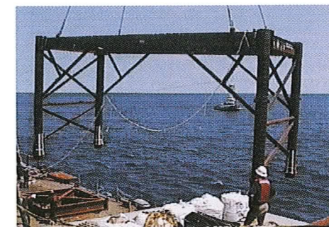
The Engine Recovery Structure (ERS) was positioned over the side of the barge and slowly lowered to the Monitor . It will be used in recovering the Monitor's engine later this year ( Monitor Collection, NOAA).
