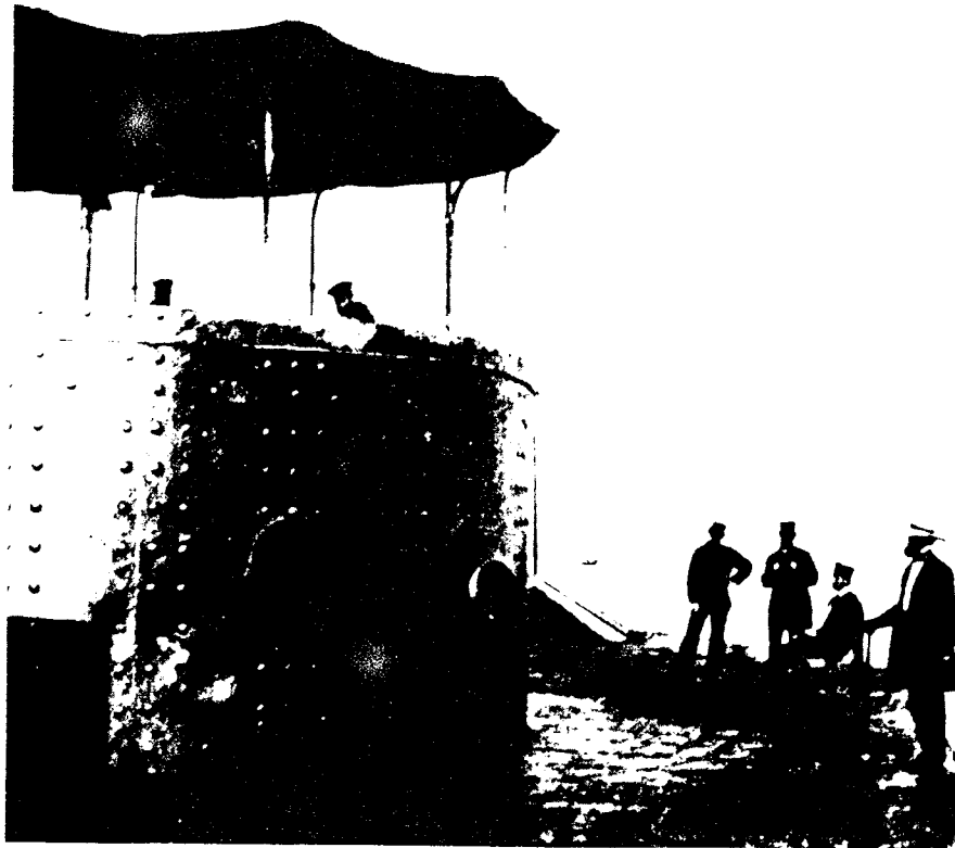
Officers examine the turret following the MONITOR's historic engagement at Hampton Roads. Dents in the turret were inflicted by the VIRGINIA during the 4 hour battle. (Courtesy of National Archives)
